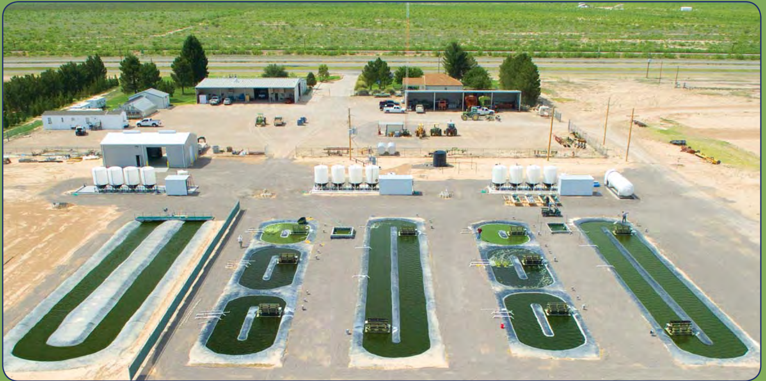
Microalgae Raceways and Cone Bottom Tanks, Pecos Algae Research and Development Facility
